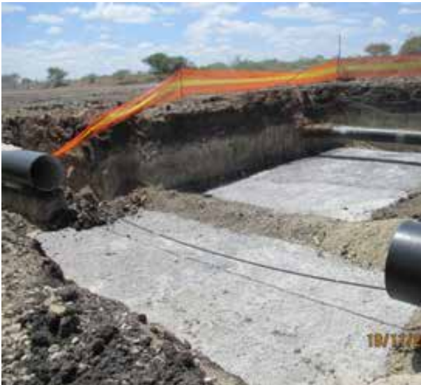
Phase 1c pipeline construction for the BPM supply
