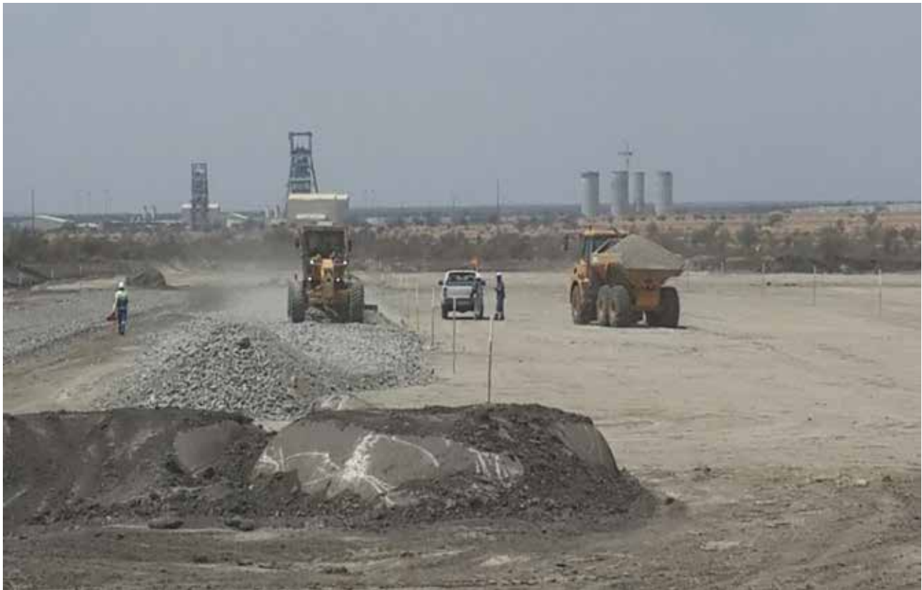
Ngwedi sub-station construction
