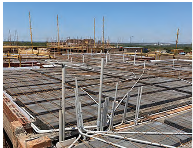
Casting of first floor rib and block slab
