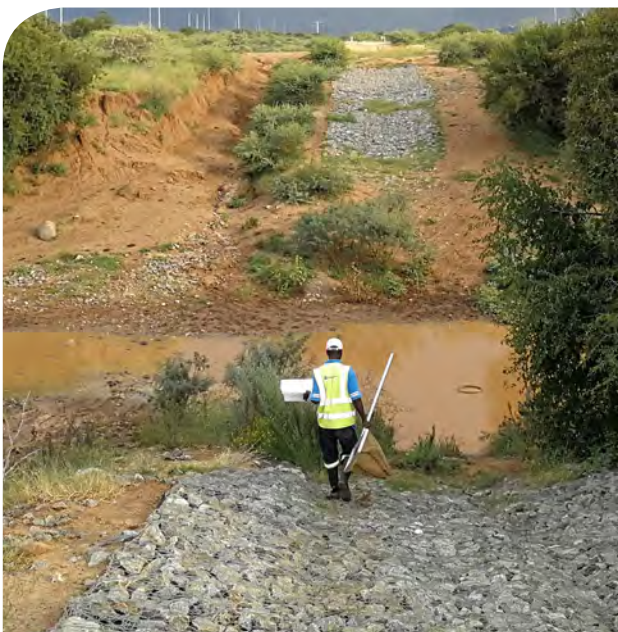
Storm water channel at Bakubung Platinum Mine.
