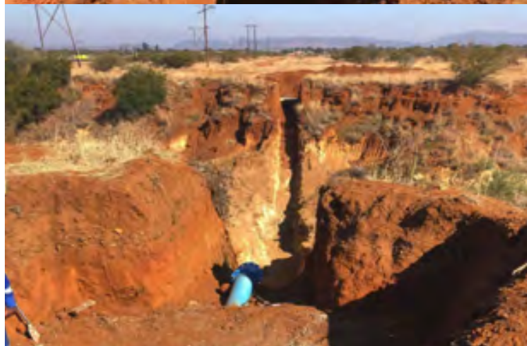
Construction of a pipeline for the water delivery infrastructure program.
