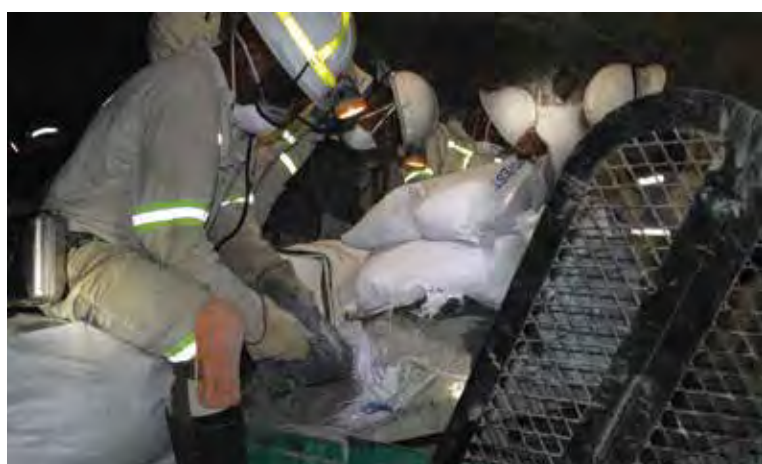
Construction of waste ore pass
