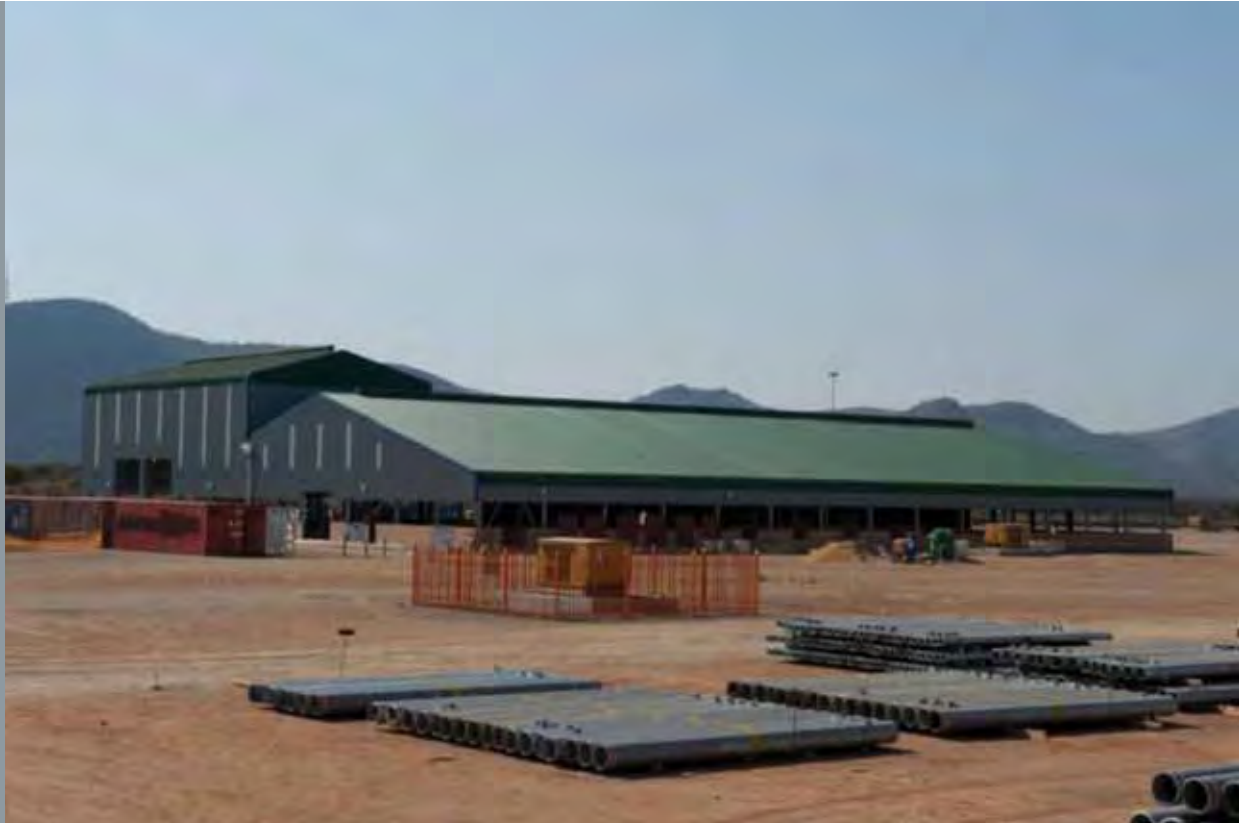
Figure 5: Main store and shaft steelwork
