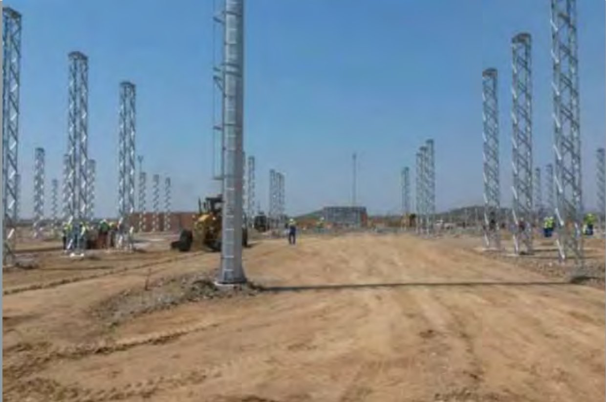
Figure 6: Ngwedi station construction (Courtesy of Eskom)
