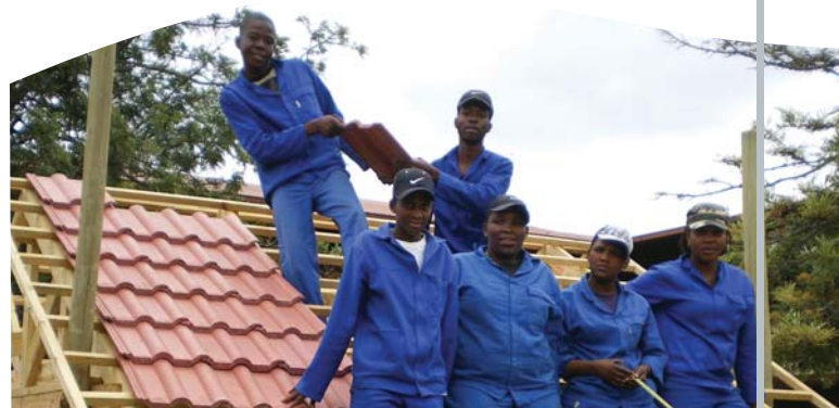
Beneficiaries participating in the Bricklaying Project
